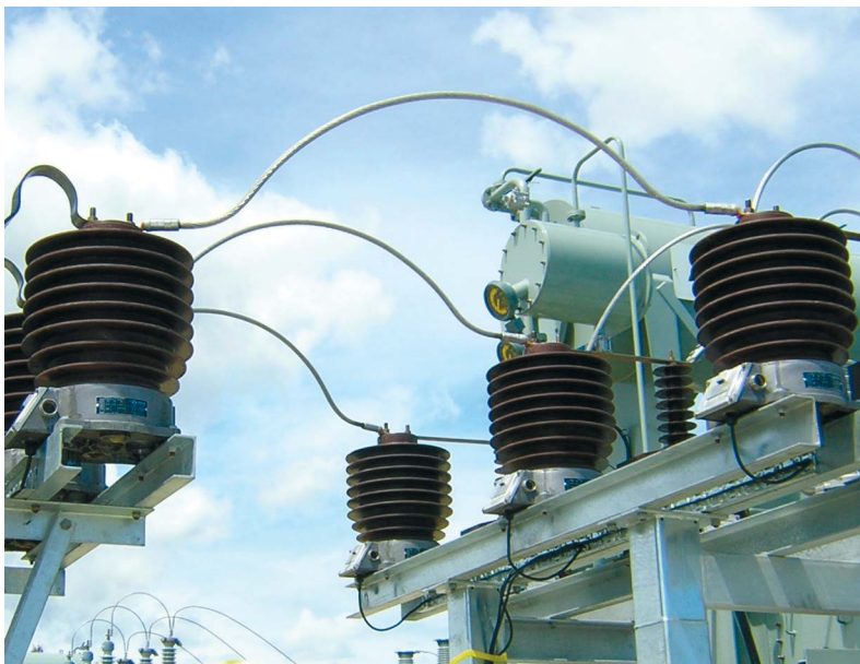
> 36 kV Current transformers (CR). Electronet Services (New Zealand).
