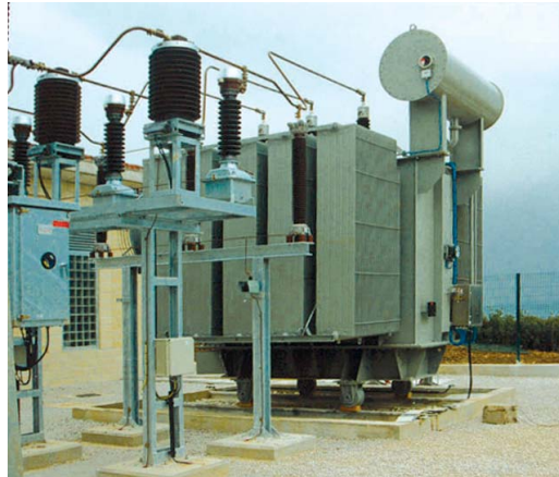
> 72.5 kV Current transformers (CX) and voltage transformers (UT) for power transformer protection. Iberdrola (Spain).
