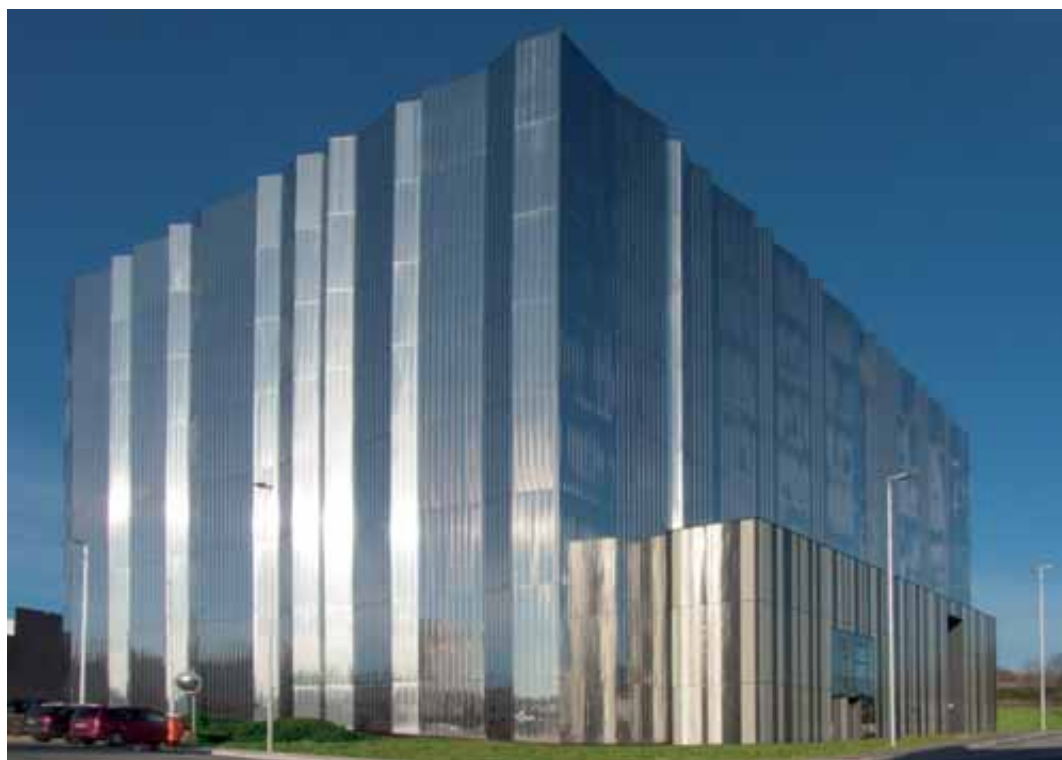
› ARTECHE new Ultra High Voltage laboratory up to 1200 kV.
